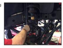
**STEP 7:** Remove lower front shock hardware and retain for reinstallation in step 14.
